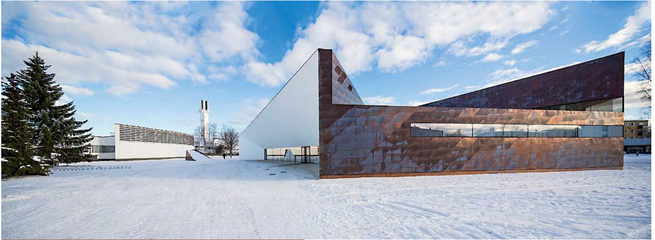
Nordic Brown products are useful to minimize hand and other construction prints which can occur for a short time after installation with “bright” standard copper.
