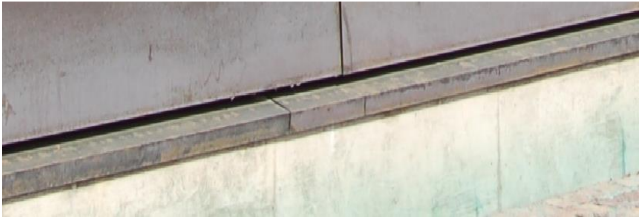
Example of copper staining on cement
