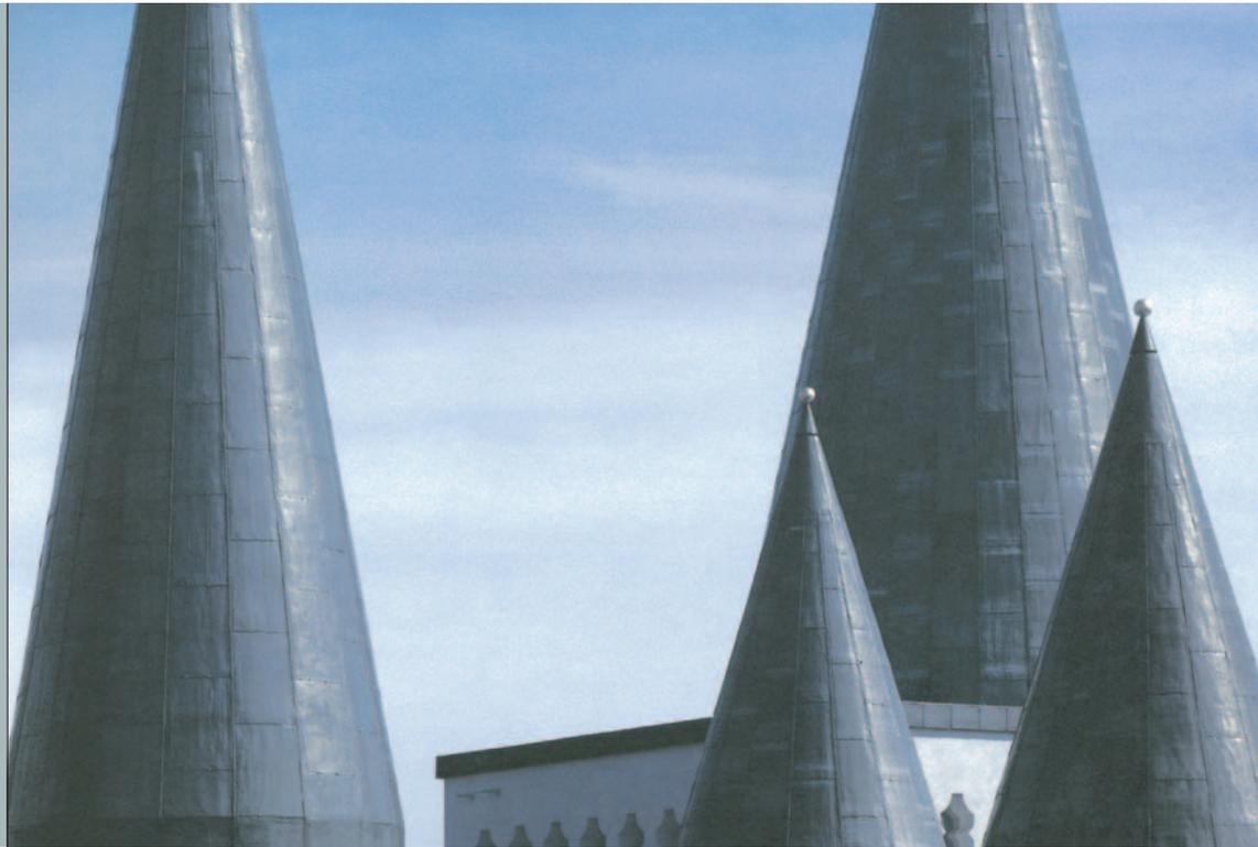
**Rolled lead Pb99.94 Cu to DIN EN 12588**
