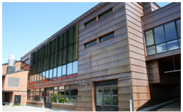
Kobberfasade, Stovner Videregående skole, Oslo
