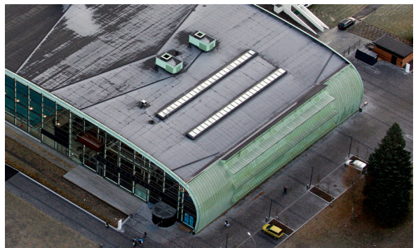
Fasade i Nordic Green Traditional, Drammensbadet
