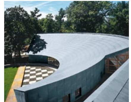
Kaplan Residence, Illinois, USA
