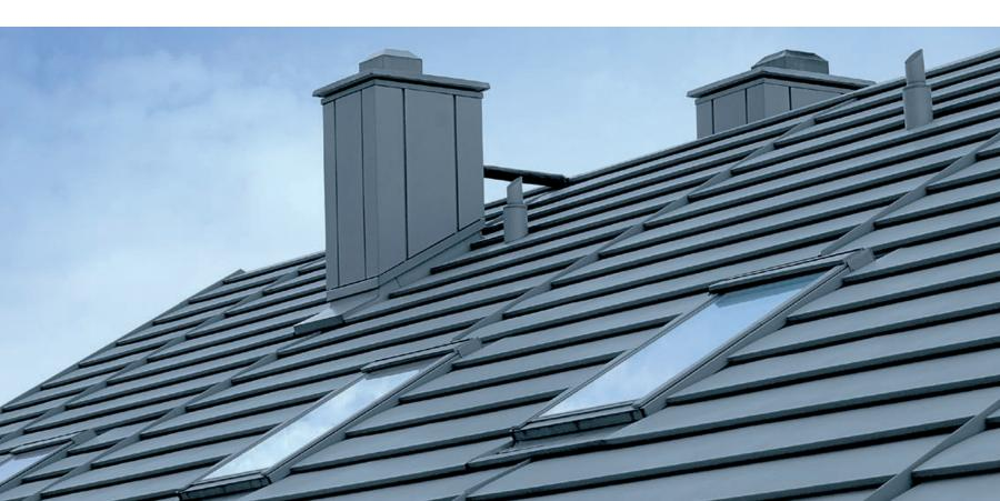
The QUICK STEP®-SolarThermie panel is one of the most economical forms of combining the advantages of an innovative metal roof with the utilisation of solar and geothermal energy. The Wetzlar solar house exemplifies this perfectly by combining QUICK STEP® SolarThermie and a heat pump for heating and hot water generation.
